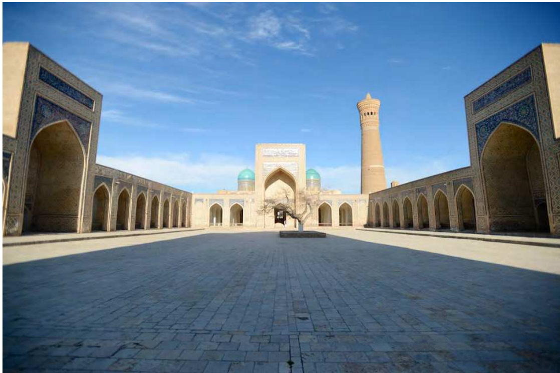
Image 10.15 Pā-i Kalān Mosque , Bukhara. The opposing four iwān face each other across the open space of the courtyard establishing the horizontal cross which also sees the main axis aligned with the qibla orientated to the Ka'bah in Mecca.
