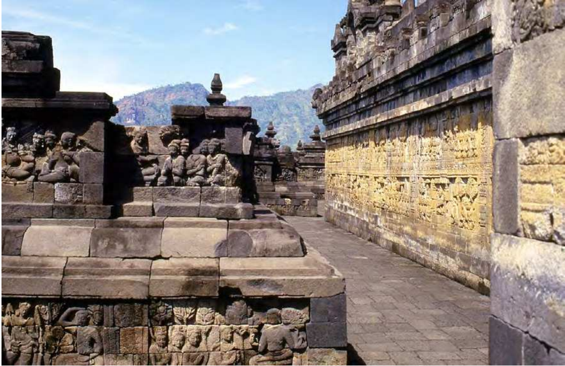
Image 7.16(a) One of the mid-level circumambulatory terraces at Candi Borobudur with carved friezes depicting the Jātakamālā on both sides of the walkway and partial glimpses of the outside view beyond.
