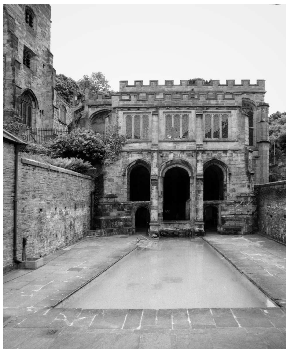
The two-storey well chapel at St Winefride's Well, Holywell: the well is inside the building and the water flows into the large outdoor bathing pool. Photo: Roger Brown.
