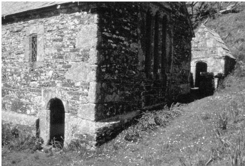
St Clether's Well and Chapel (1990). To the right is the holy well (or the upper well); in the centre is the east end of the chapel; and at bottom left is the lower well where the water emerges from the chapel.
