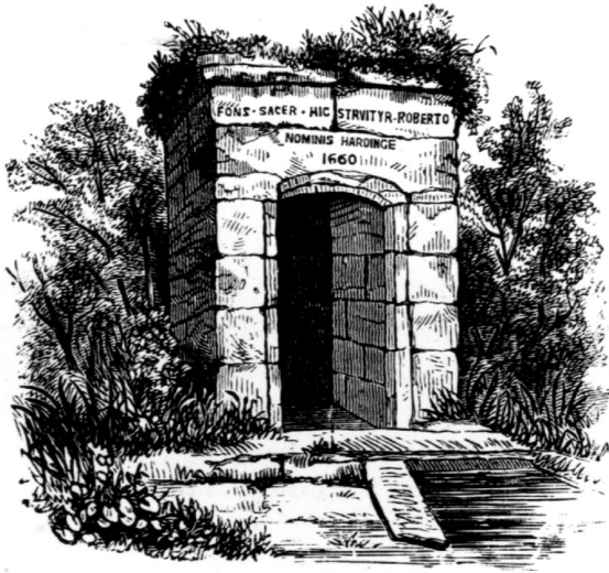
The holy well at King's Newton before the first arch collapsed.
