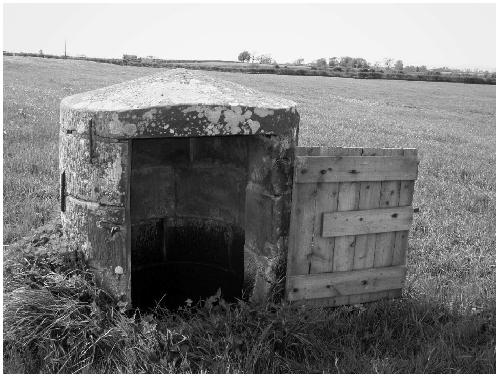
The door of St Mungo's Well near Bromfield church is normally kept secured for safety reasons: there is a deep well inside the small well-house. Photographed in 2007.
