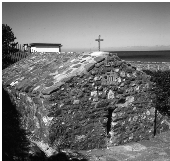
The solid stone building which now covers Ffynnon Drillo, photographed in 1988. The well is in the floor just behind the east wall facing the photographer.
