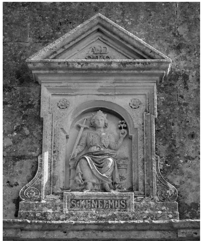
Top: The well-house built over St Kenelm's Well, Winchcombe; photographed in 2006.
