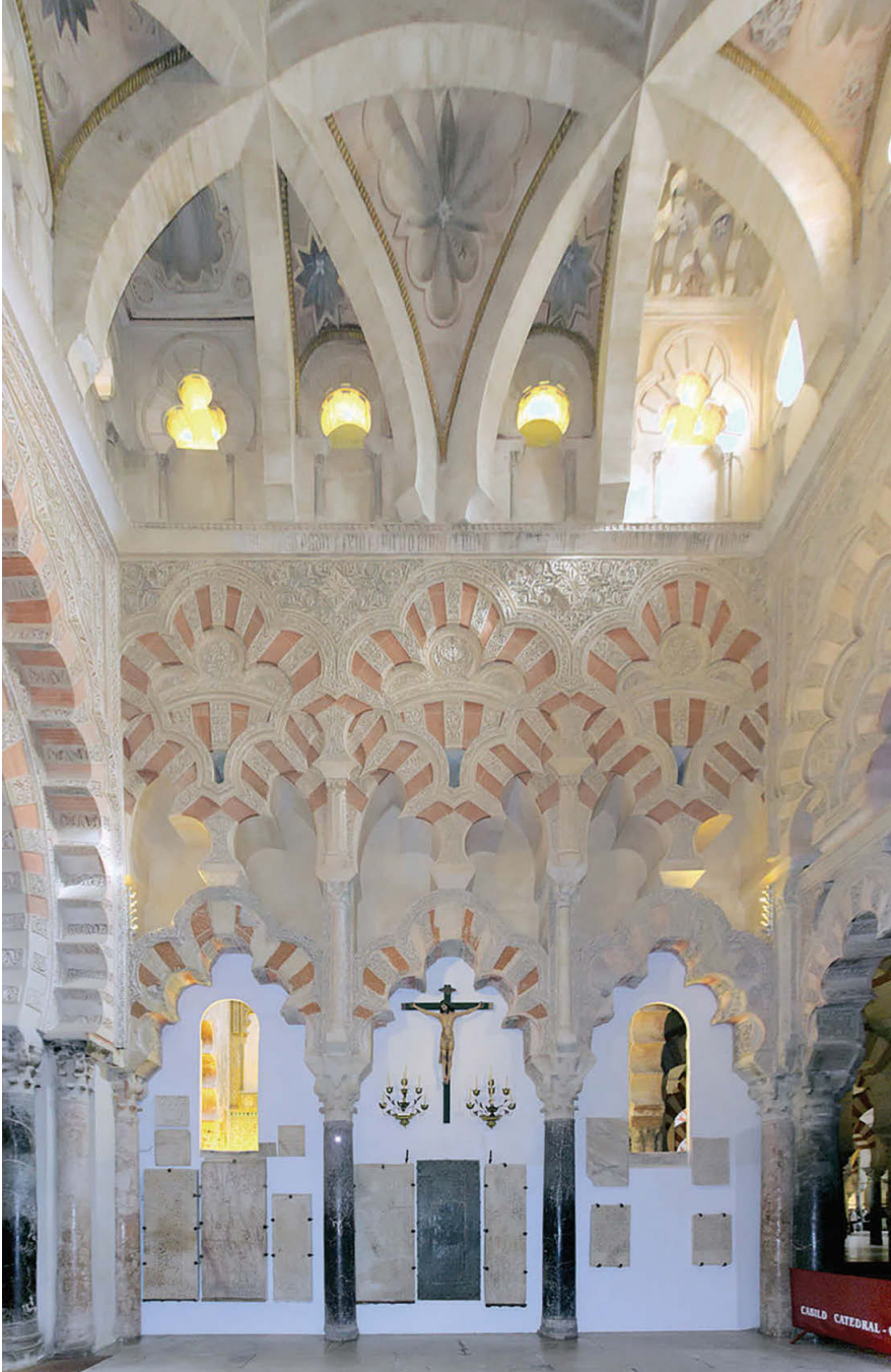
Ribbed cross vaulting of the Capilla de Villaviciosa, Cordoba Mezquita, a masterpiece of tenth-century geometry that has never needed structural repair.
