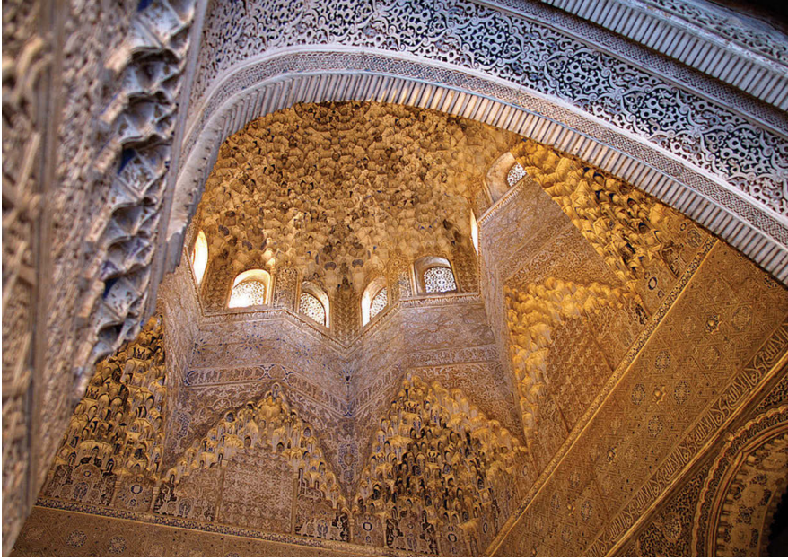
MUQARNAS, HONEYCOMB, STALACTITE OR MOZARABIC VAULTING IN THE HALL OF THE ABENCERRAJES, ALHAMBRA
