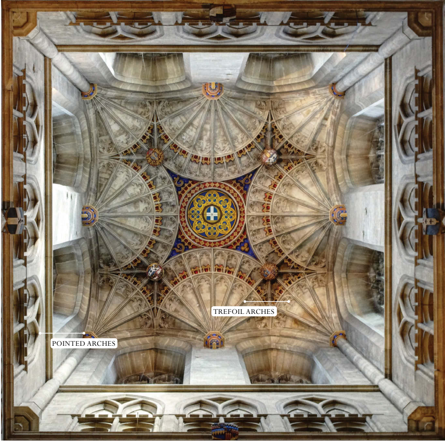
CANTERBURY CATHEDRAL, FAN VAULTING OF THE CROSSING
