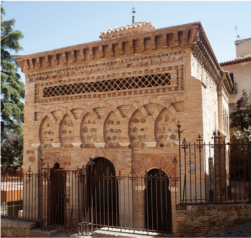
The brick-built miniature Bab al-Mardum Mosque in Toledo was modelled on the tenth-century extension to the Cordoba Mezquita, copying its arches and its ribbed vaulting. Today it is the church of Cristo de la Luz.
